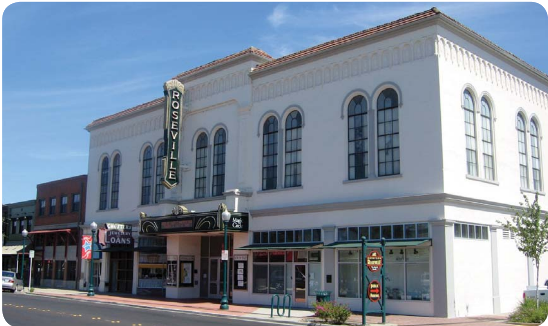
The Magic Circle Theater has both an electronic programmable sign and a vertical marquee sign
