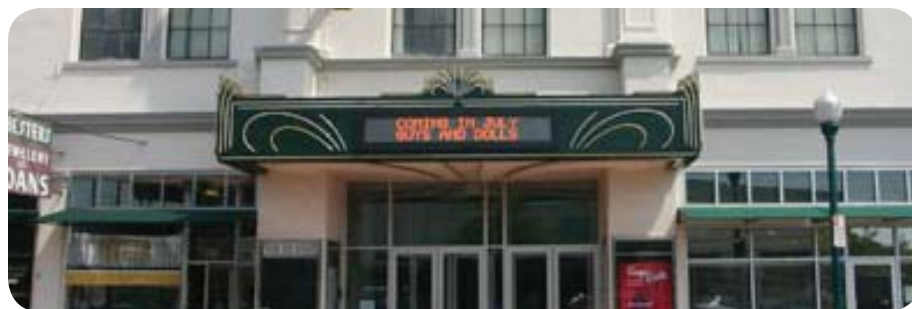
Figure 8.12.1 The Magic Circle theatre sign is an example of a Programmable Electronic (PE) sign
